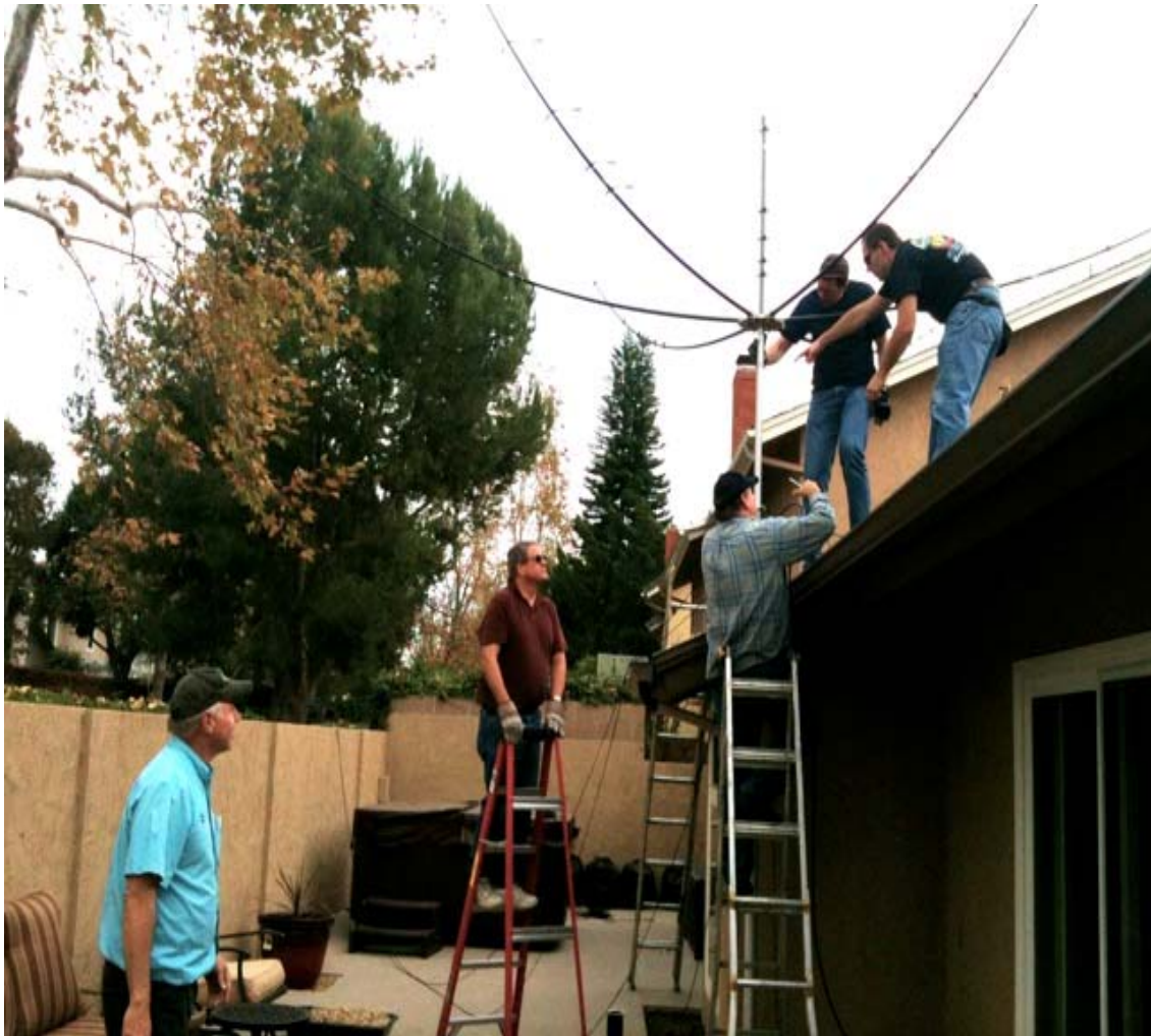
Antenna is mounted onto the mast (from left: N8AE, K6GEP, AE6RS, KR6J, W6UX)
