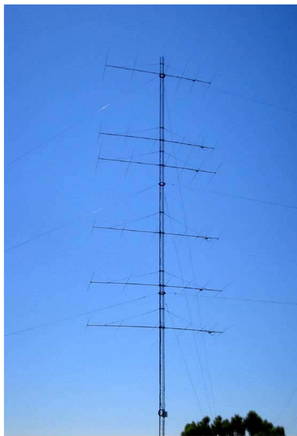
Fig 2 – One of the many rotating towers at the W6BH site.
