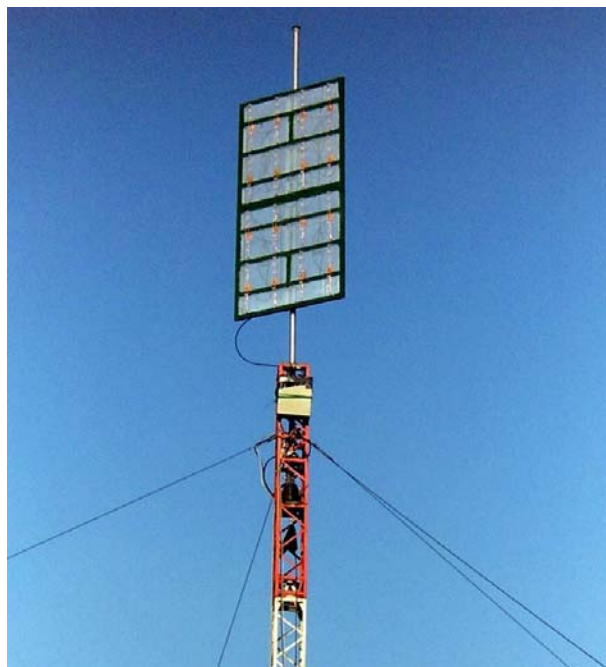
Figure 6 – The Large 6-loop panel array by HA5IW mounted up on the Tower. (Courtesy of Paul G8GML)
